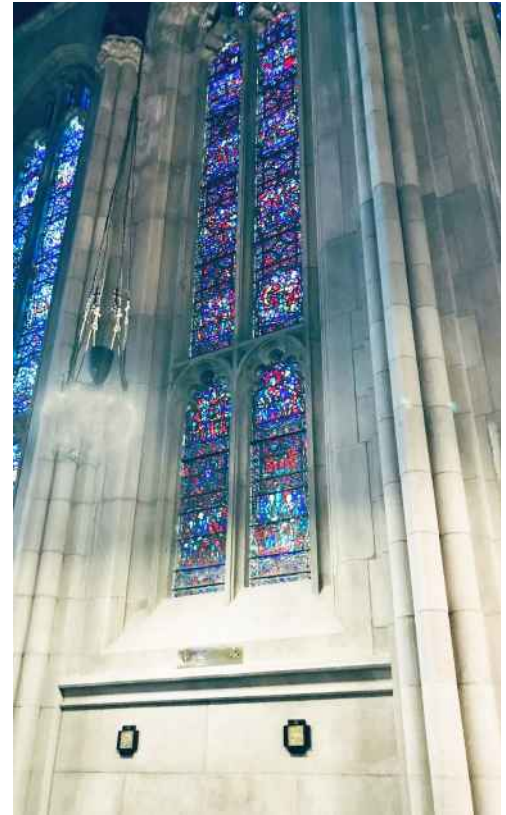
The 12 pane window restored →
